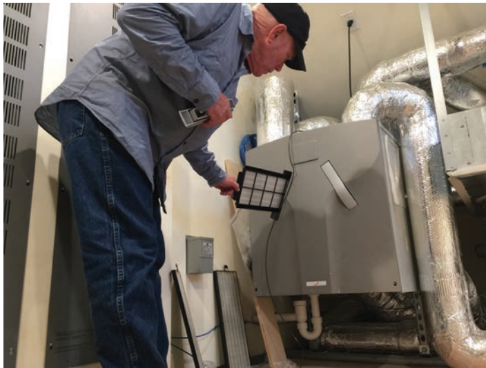
Builder Jeff Adams inspects an air filter for the Zehnder heat recovery ventilator serving the home (above left). A smoke detector tied into the Zehnder controls at the system's fresh-air intake port (above right) is wired to shut the fans down and close a damper if smoke from a wildfire begins to enter the system.
