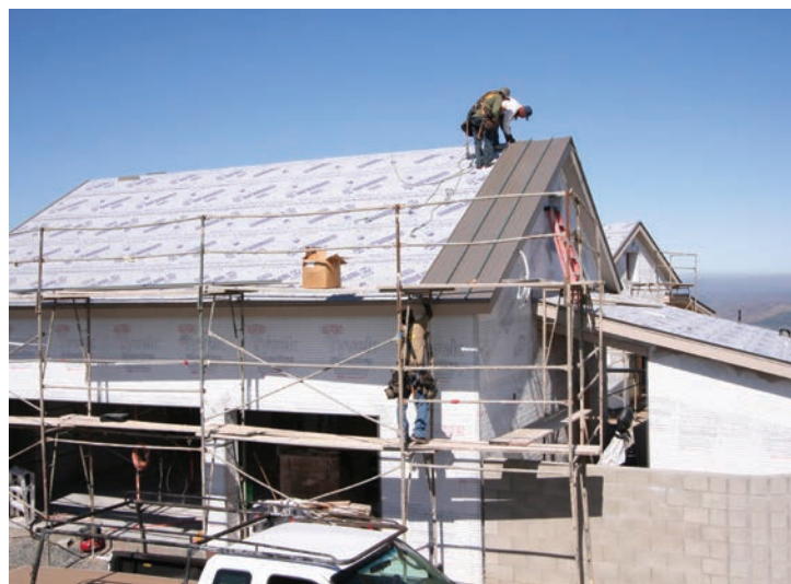
Carpenters apply 6-inch SIPs to the roof frame (top). The roof sheathing under the SIPs has already been air-sealed with fluid-applied membrane. Above, roofers install steel roofing panels on top of synthetic roofing underlayment.
