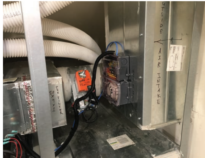
Builder Jeff Adams inspects an air filter for the Zehnder heat recovery ventilator serving the home (above left). A smoke detector tied into the Zehnder controls at the system's fresh-air intake port (above right) is wired to shut the fans down and close a damper if smoke from a wildfire begins to enter the system.
